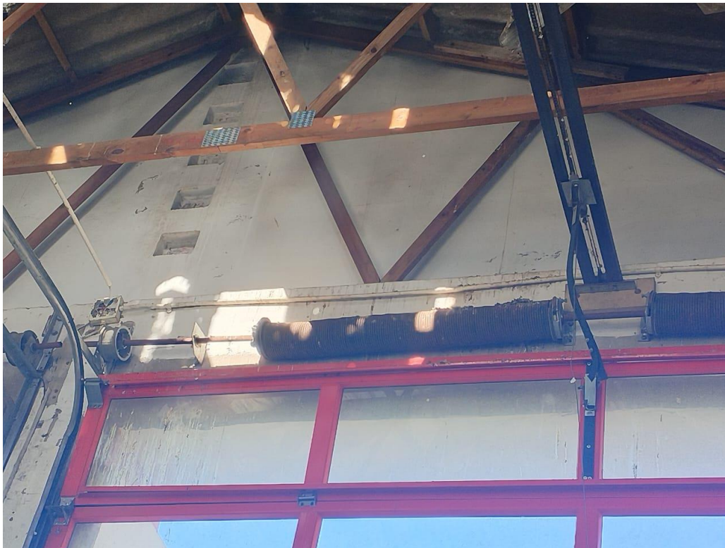
Engine Bay Doors Cable Missing
