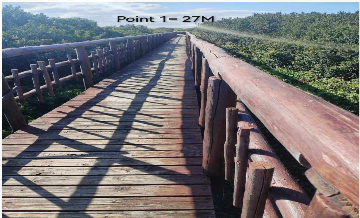
Point 1: Replacement of decking and vanishing with Mahogany colour. Dimensions of the decking – (W x123cm) (L x 27m)
