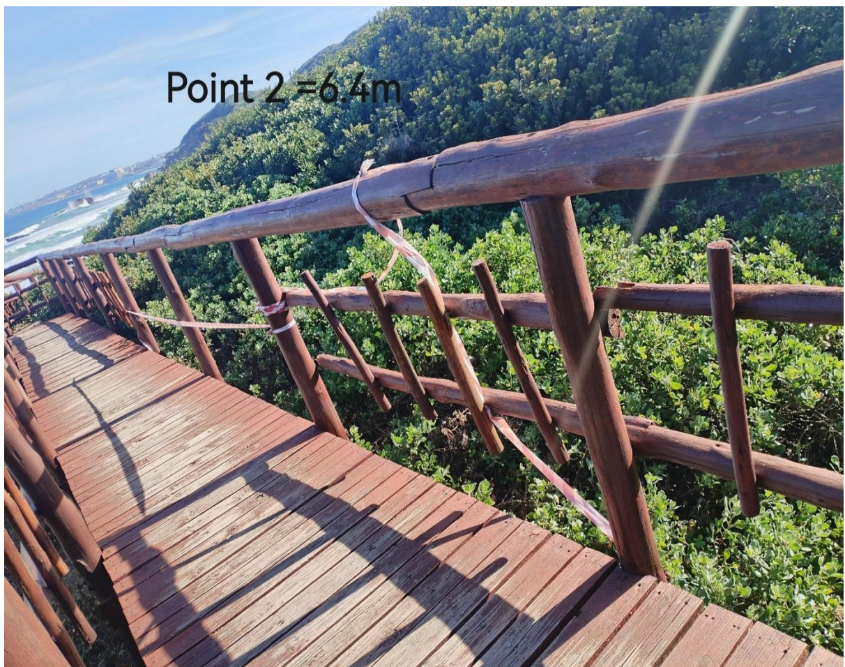
Point 2 (icon site): Replacement of rails and vanishing using Mahogany colour
