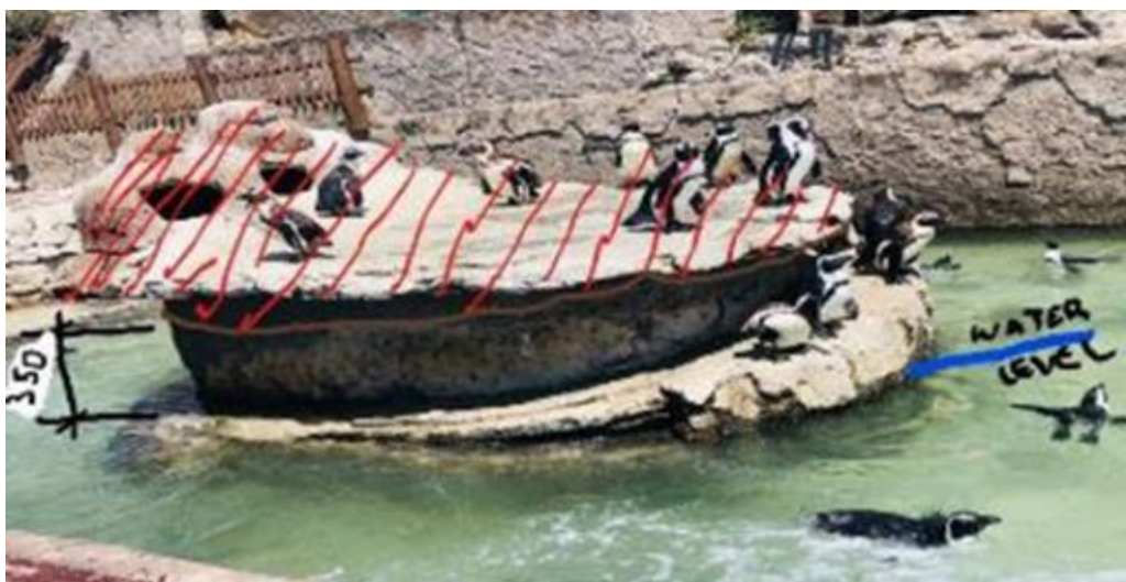
Photo 3 : Centre Piece to be demolished to 350mm above the existing water line
