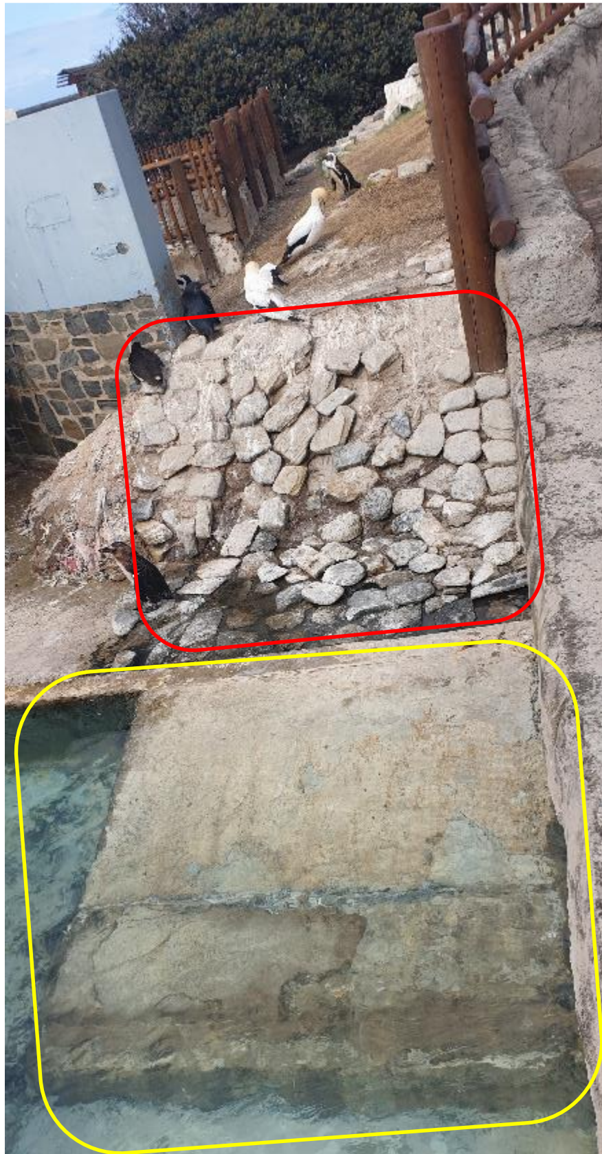
Photo indicating Concrete slip way to be prepared and resurfaced with similar plaster coating 25 – 30 mm thick. (Indicated in yellow rectangle). The Stone pitched causeway to be repaired. Loose stones to be repaired and adhered. To be grouted with epoxy as specified by Supplier. (Red rectangle)
