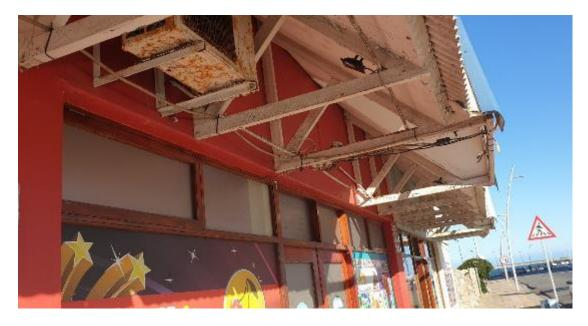
The photo above indicated the Roof Timber Structure of the Covered Patio. Note that the timber will have to be sanded down, treated with Timber Primer and painted two coats of suitable paint as per specification supplied at briefing.
