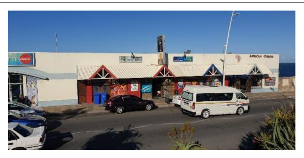
Note the Covered Patio. The roof structure consists of a mix of (1) Fibre Cement/Asbes Roof sheets to be painted in same colour, (2) Section replaced with Corrugated Iron roof sheets. Same colour as the Fibre Cement Roof Sheets. Note that the preparation will differ.
