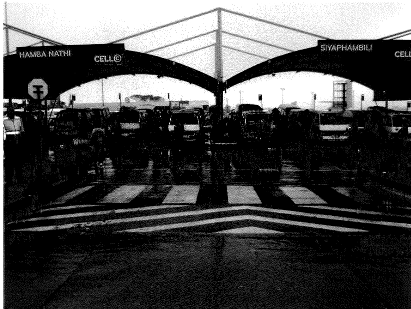
Figure 2: Ramps for disabled passengers at the Highway Taxi Rank, Mdantsane
