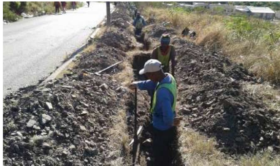
Cable installation
