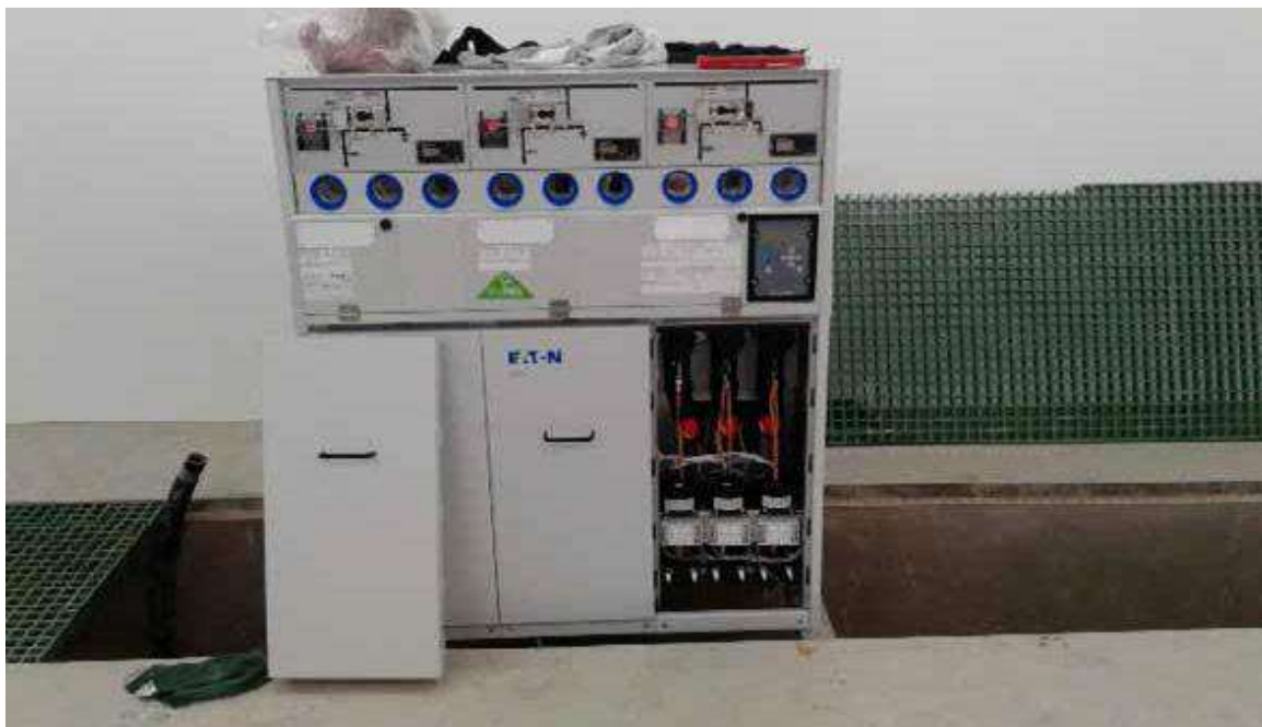
Installation of New Switch Gear
