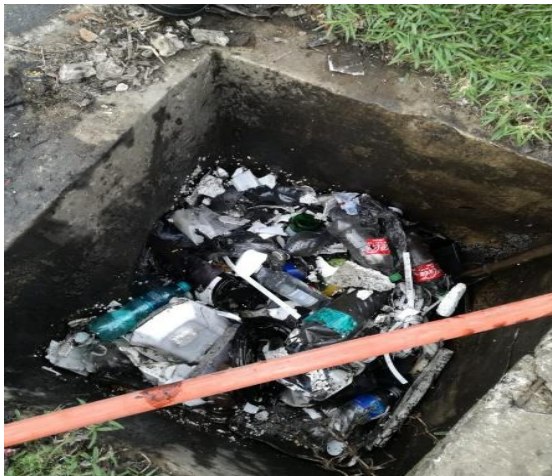
Waste found in stormwater drainage infrastructure
