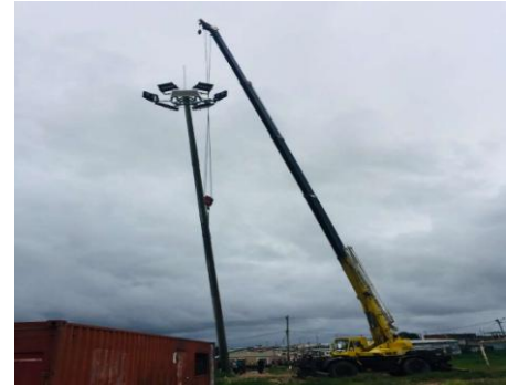
Mast being erected
