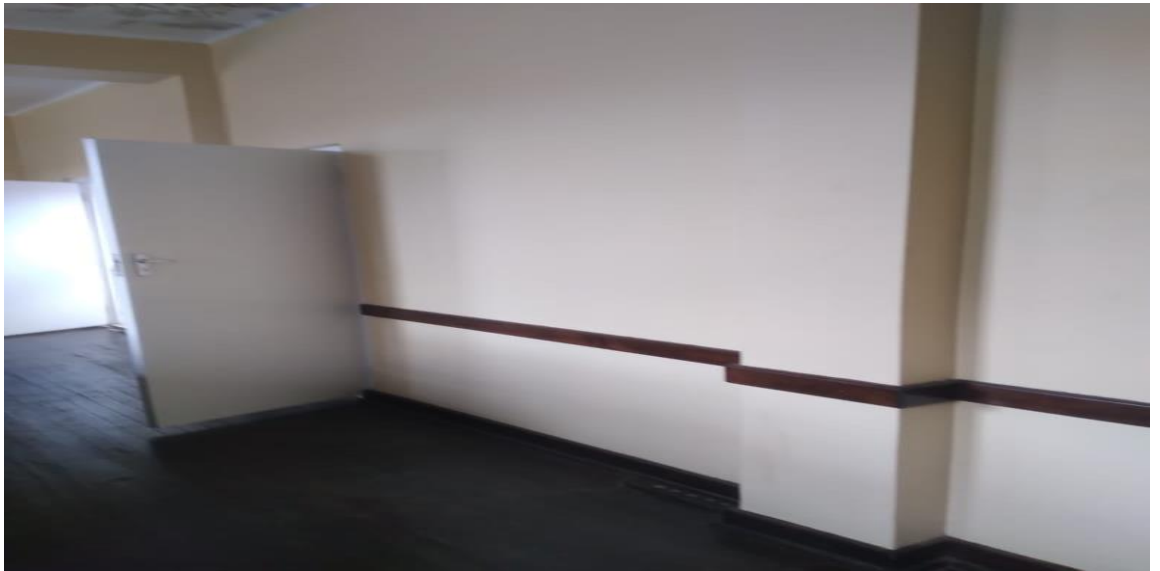
Figure 117: Greenfields refurbishment cont'
