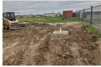
Backfilling & compacting done
