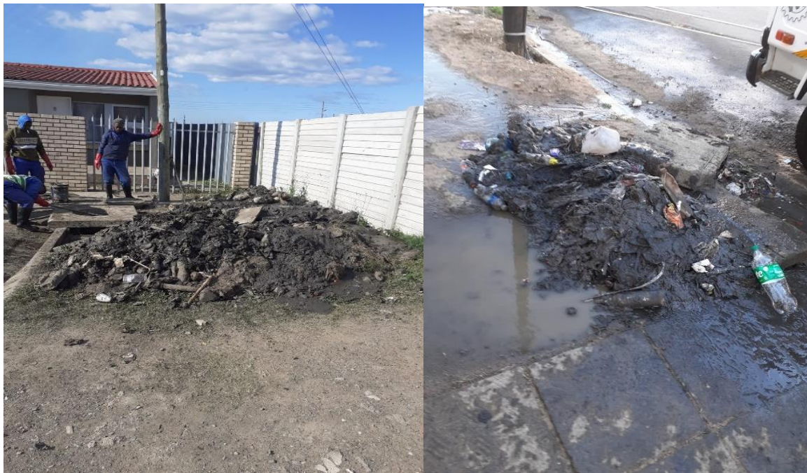
Figure 27: Waste typically found in stormwater system
