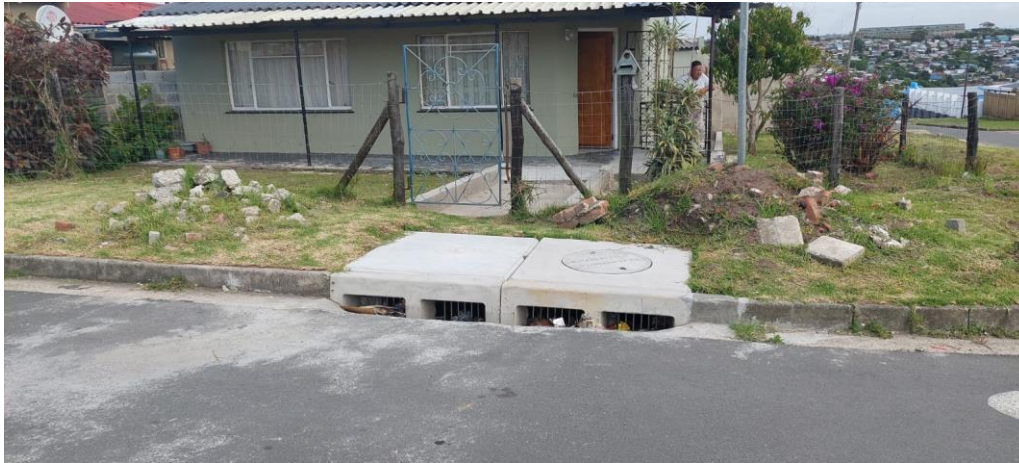
Figure 26: (a) and (b) new kerb inlets
