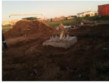
Backfilling & compacting almost done
