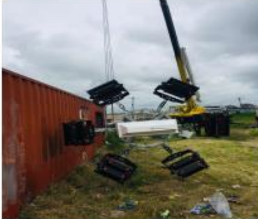
Mast spitter box & lights installed
