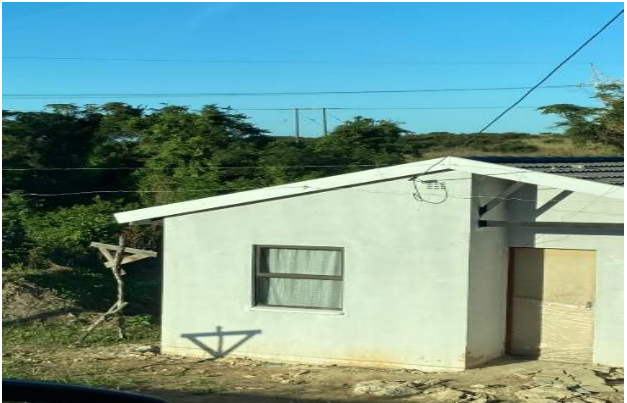
Figure 18: Service connection entering dwelling
