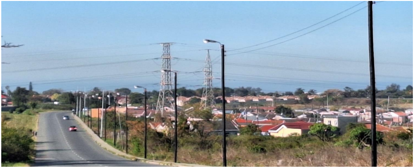
Figure 11: Street lighting in BCMM
