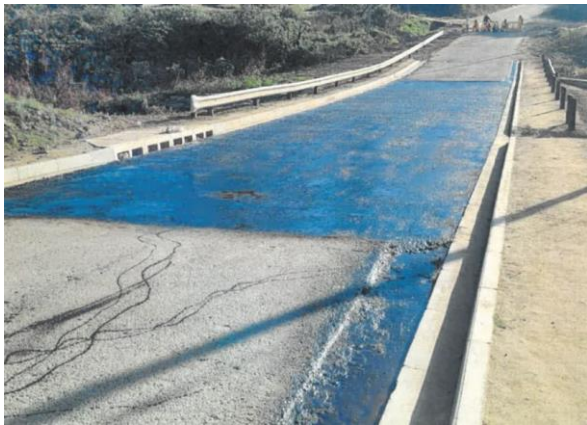
Figure 31: Potsdam Culvert Flood rehabilitation: clearing and repairing the existing inlet and outlet structures
