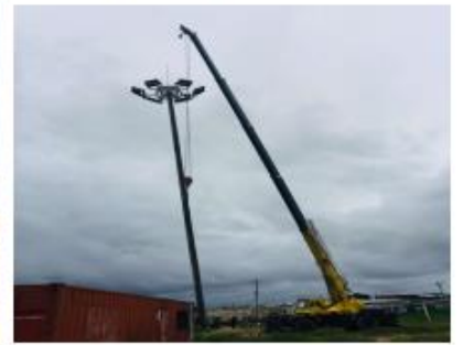
Mast being erected
