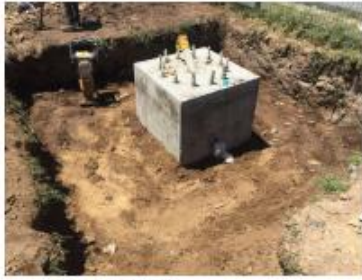
Backfilling & compacting
