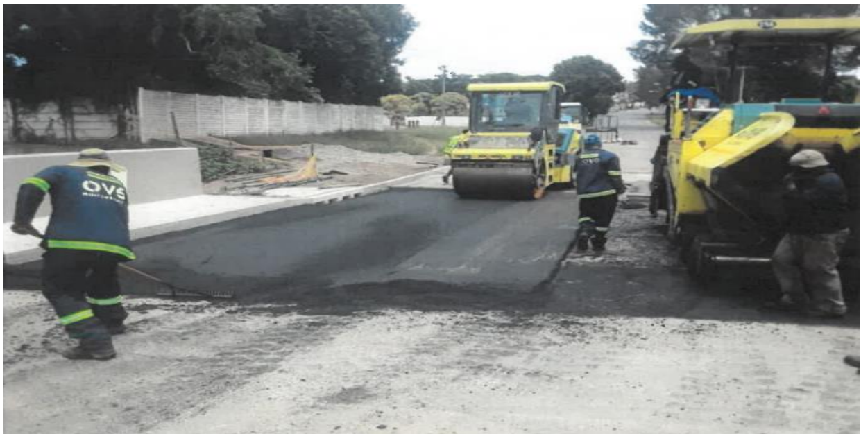
Figure 30: Pottinger Street Bridge refurbishment – new deck
