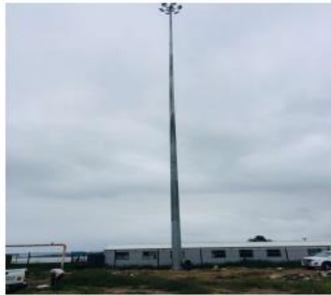
Highmast completely erected
