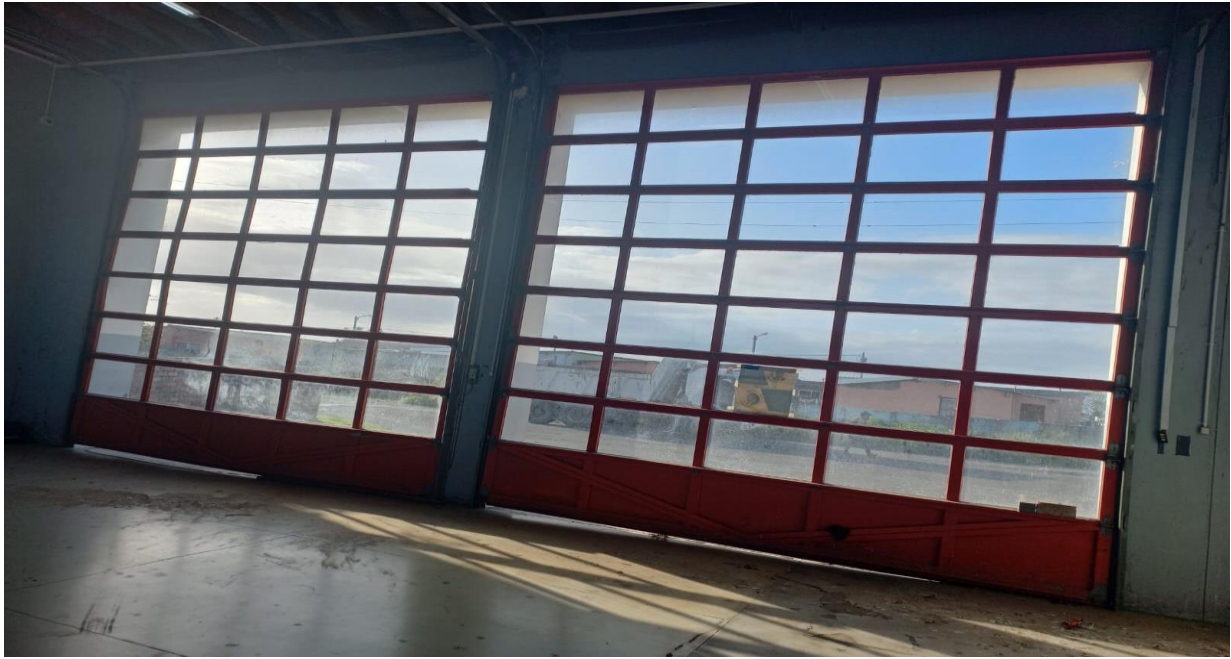
Figure 115: Gompo engine bay doors
