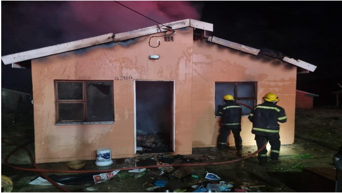
Figure 106: House fire May 2023
