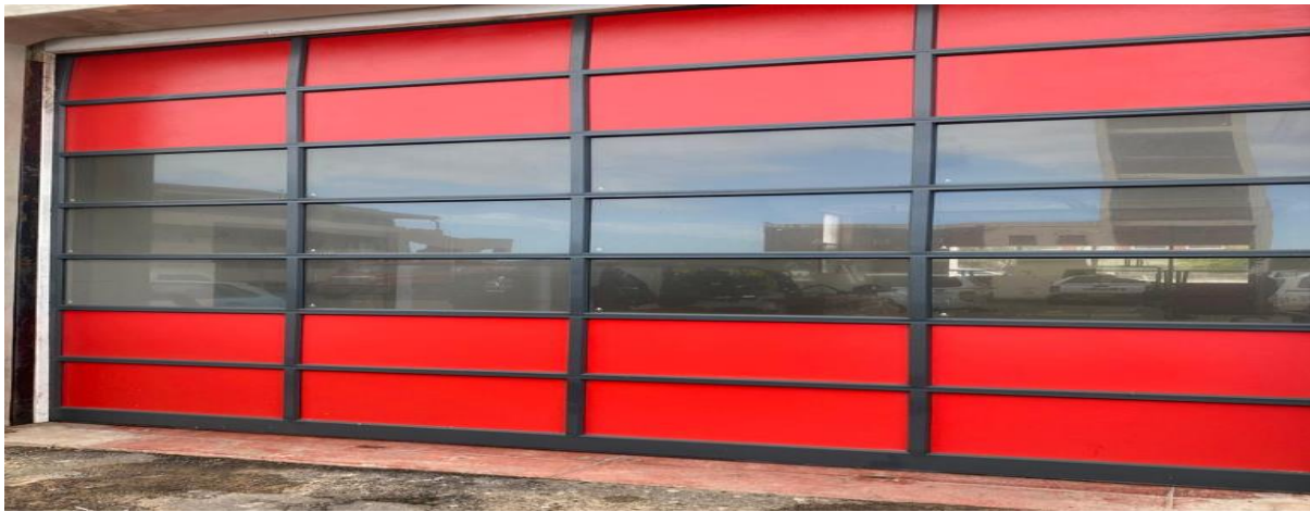
Figure 113: New engine bay doors – Fleet Street Fire Station
