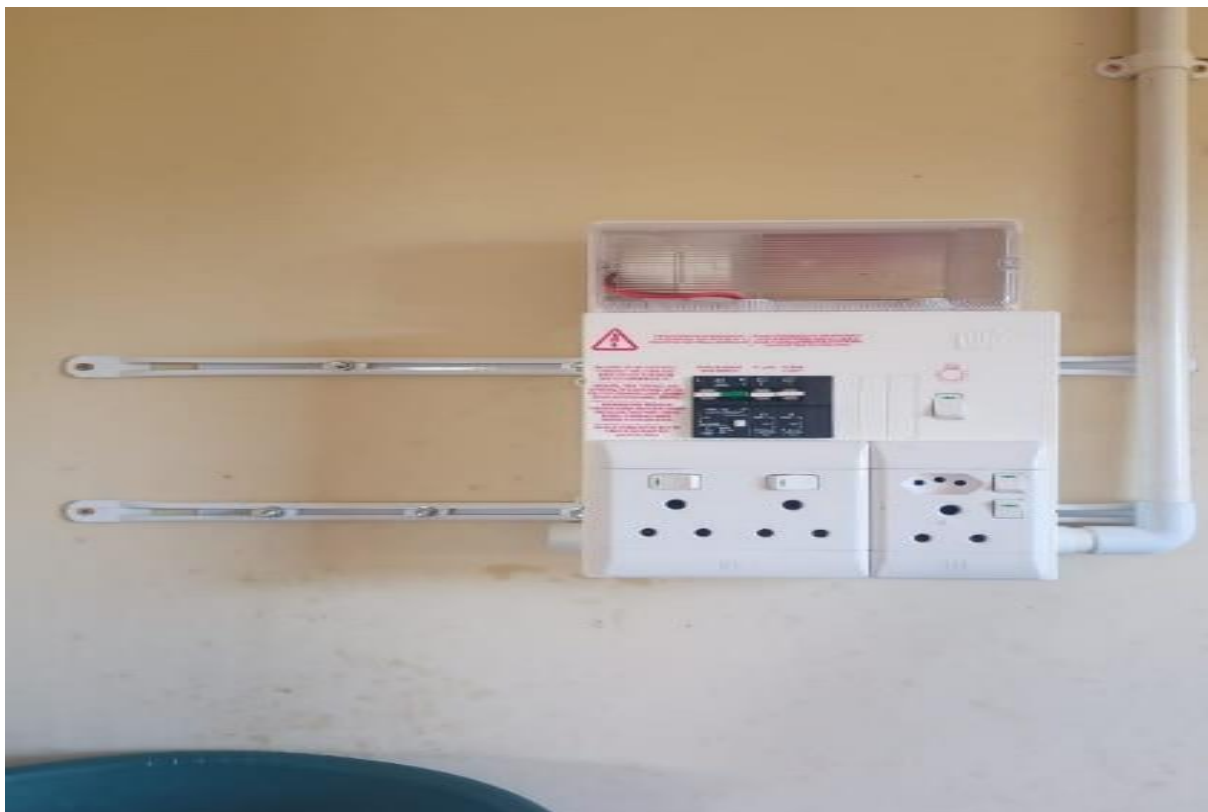
Figure 16: Ready board installation on rails
