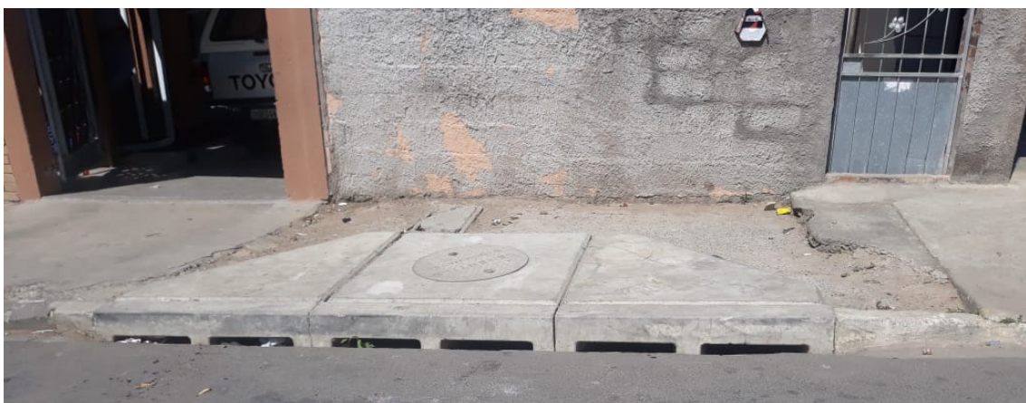
Above: New Kerb Inlets
