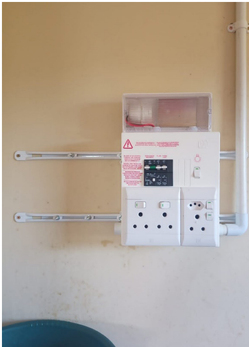
Ready board Installation on rails
