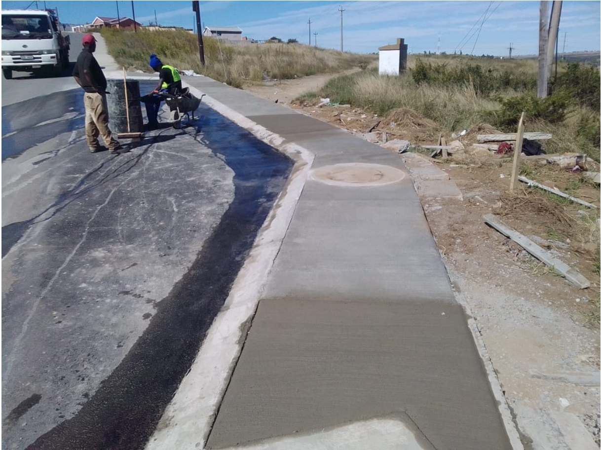
Completed Construction of 3 Taxi/ Bus Embayment's in Sweetwaters & Mdantsane
