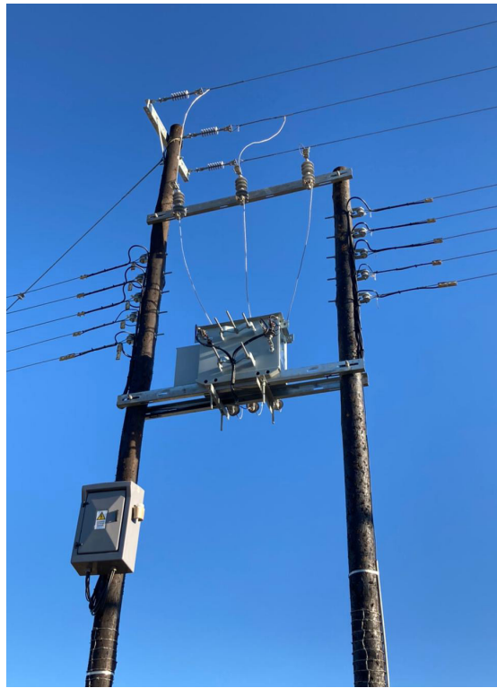
Transformer/ Network construction
