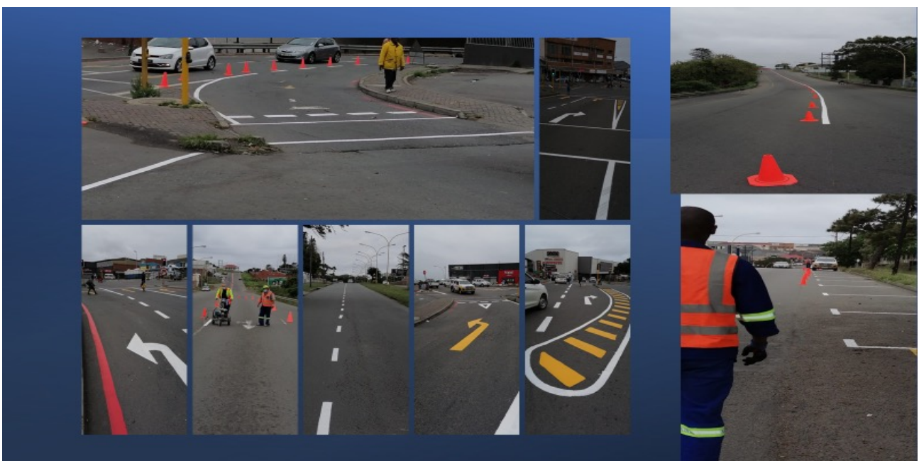
Figure 1 Various Road markings for 2021-2022 were done.
