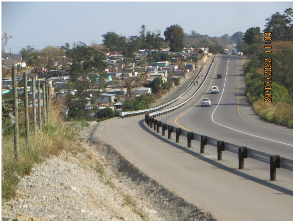
Mdantsane Access Road 2km of Road Widening
