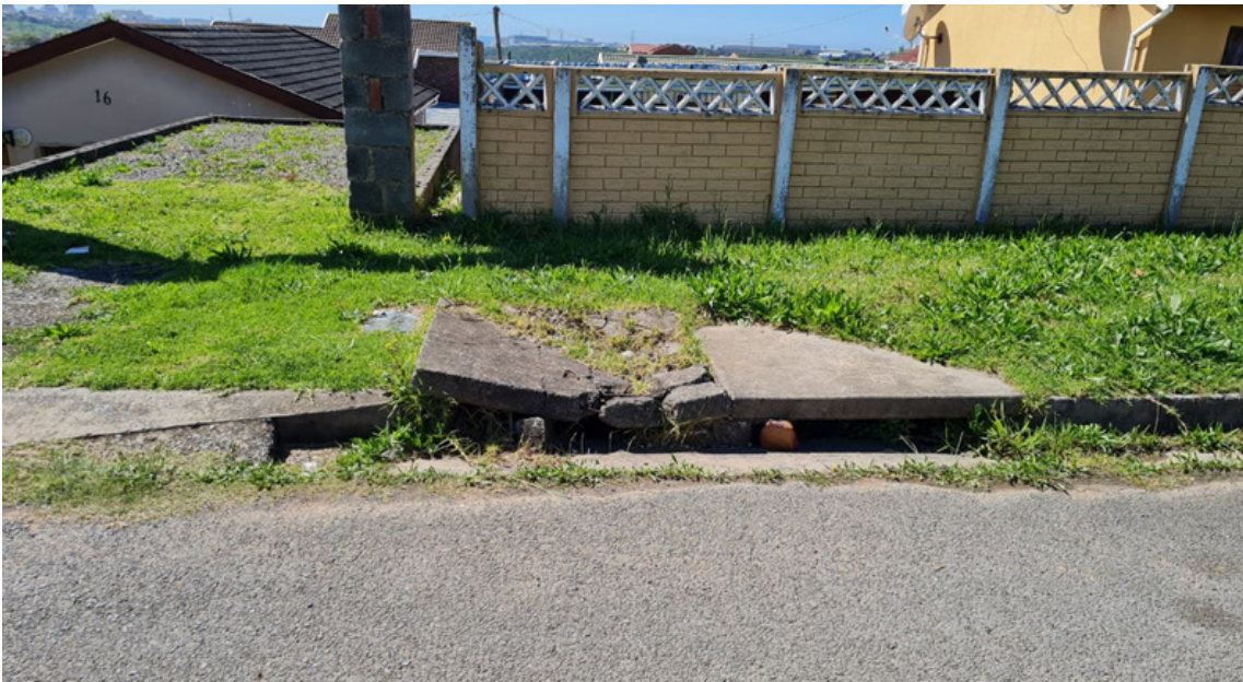
Above: Damaged Kerb Inlets
