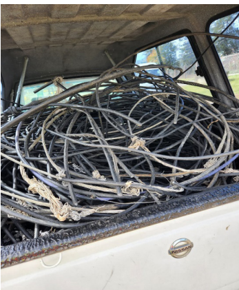
Recovered stolen cable from illegal connections
