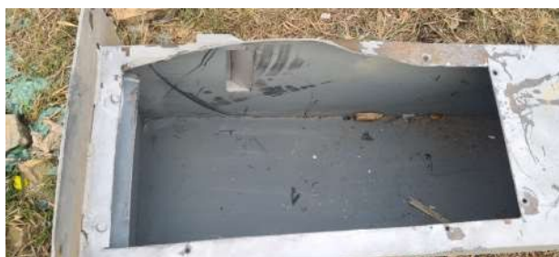
Pole base vandalized and equipment stolen out of it in KWT
