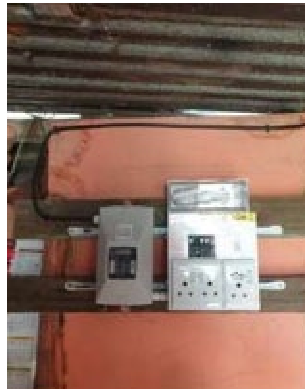
Ready board/Meter Installation on rails
