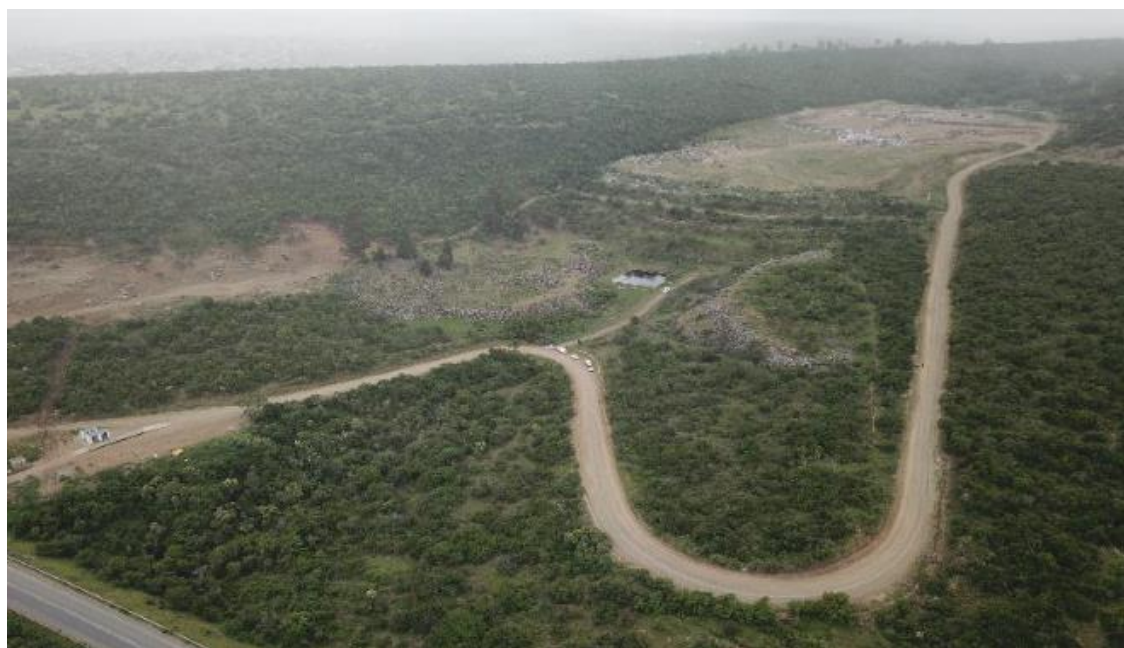
Figure 12: King William's Town Landfill Site: Entrance and Weigh bridge bottom left, Leachate pond centre, waste mass upper right quarter, working face in centre of waste mass
