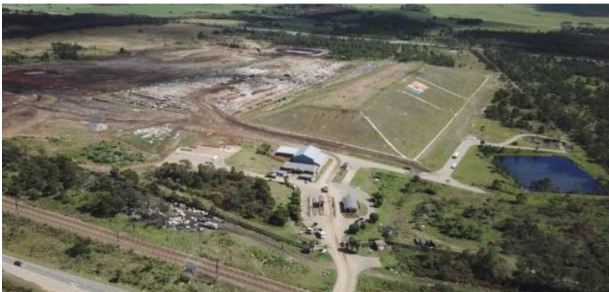
Figure 10: Roundhill Landfill Site - Leachate pond right, followed left to right by Cell 1 (covered), Cell 2 (current), Cell 3 under construction, cell 4 will join Cells 1 and 2. Railway line in foreground, highway in background with weighbridge and
