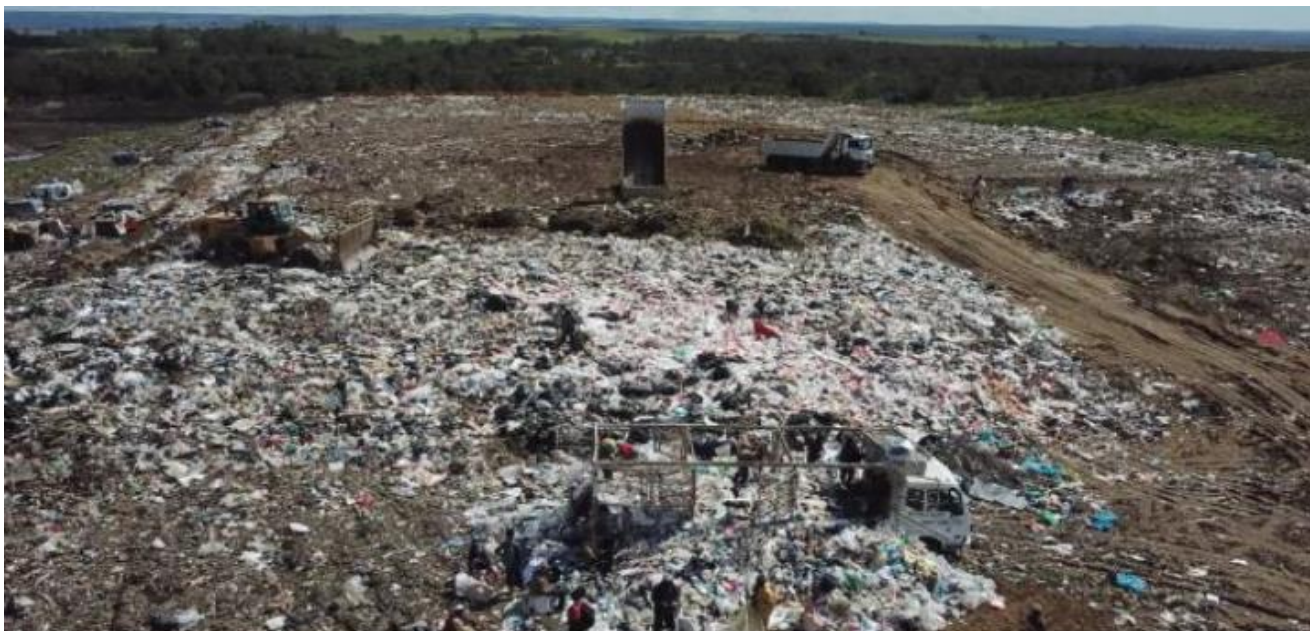
Figure 11: Working face of Roundhill Landfill. Green Waste "cover material" from Beacon Bay Green Waste Transfer Station deposited in far ground; cage truck unloading of MSW in foreground; landfill compactor left upper-middle.
