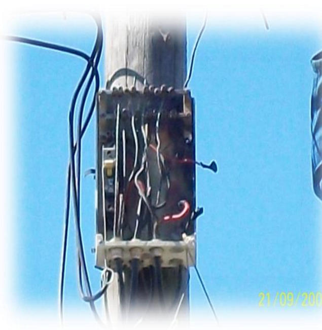
Damaged Equipment due to illegal connections
