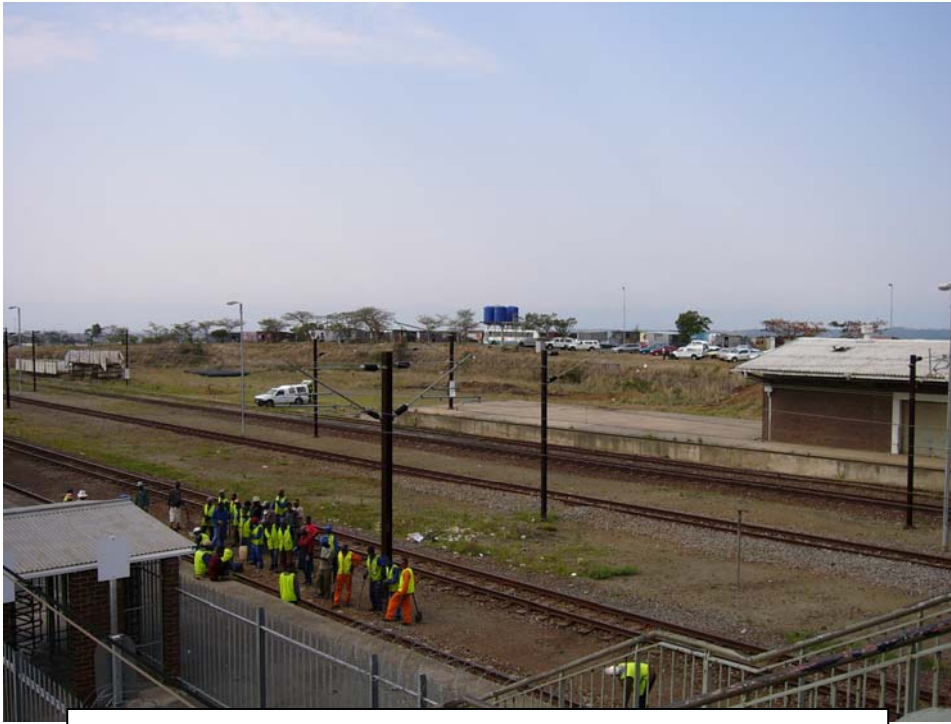
A: View of railway station area where ground and groundwater contamination is probable.
